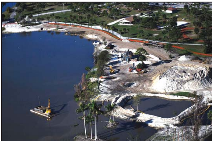
In this aerial view of the project in Florida, a mechanical dredge is digging into a barge. The Del separator system is visible on shore about midpoint in the photo. Almost 80,000 cubic yards of material was dredged and dewatered in the course of the project.
