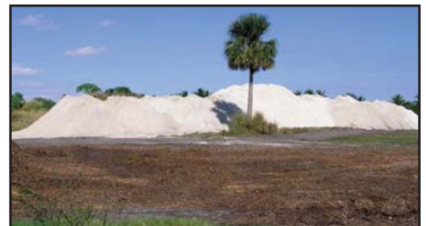
Stockpiled material to be used in the park. The dredge and dewatering system processed about 80,000 cubic yards of sand, at times at a rate of 100 cubic yards per hour.
